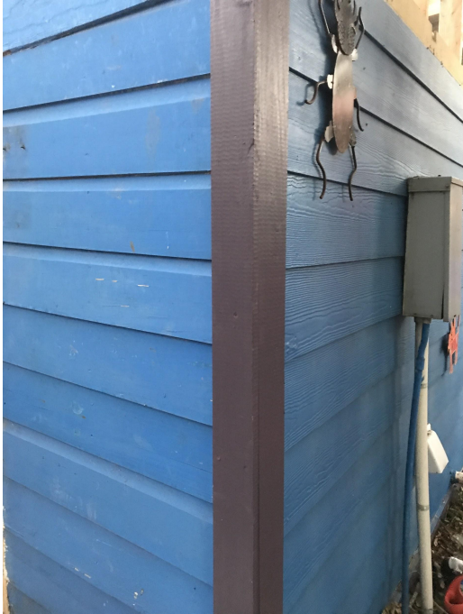
Current sides with hardboard and wood to be replaced
